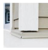
1/4" 1/4" above flashing: Flashing is imperative, but maintain a 1/4" gap for a capillary break.
