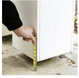
2" Install 2" above porches, roofs, etc: 2" breaks are crucial on the porches, roofs and all flat surfaces (patios, decks, etc).
